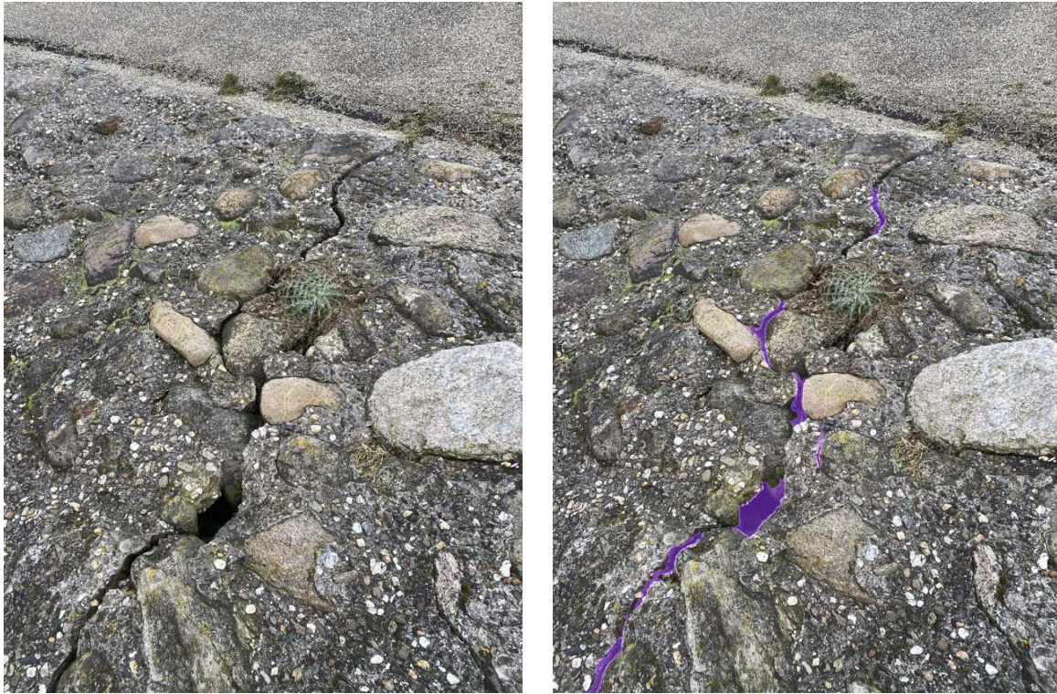
Figure 2. Crack detection using an AI algorithm on a traditional dike inspection photo (photo taken by Veenstra, March 2025; the purple overlay, which is the pixel-wise prediction of location of cracks, is generated using a model trained via a CNN-based crack detection model 1 ).
