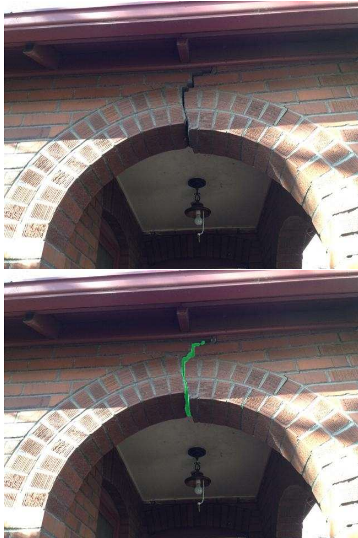
Figure 2. An example crack prediction by the proposed method (the green shade is the crack prediction overlay)
